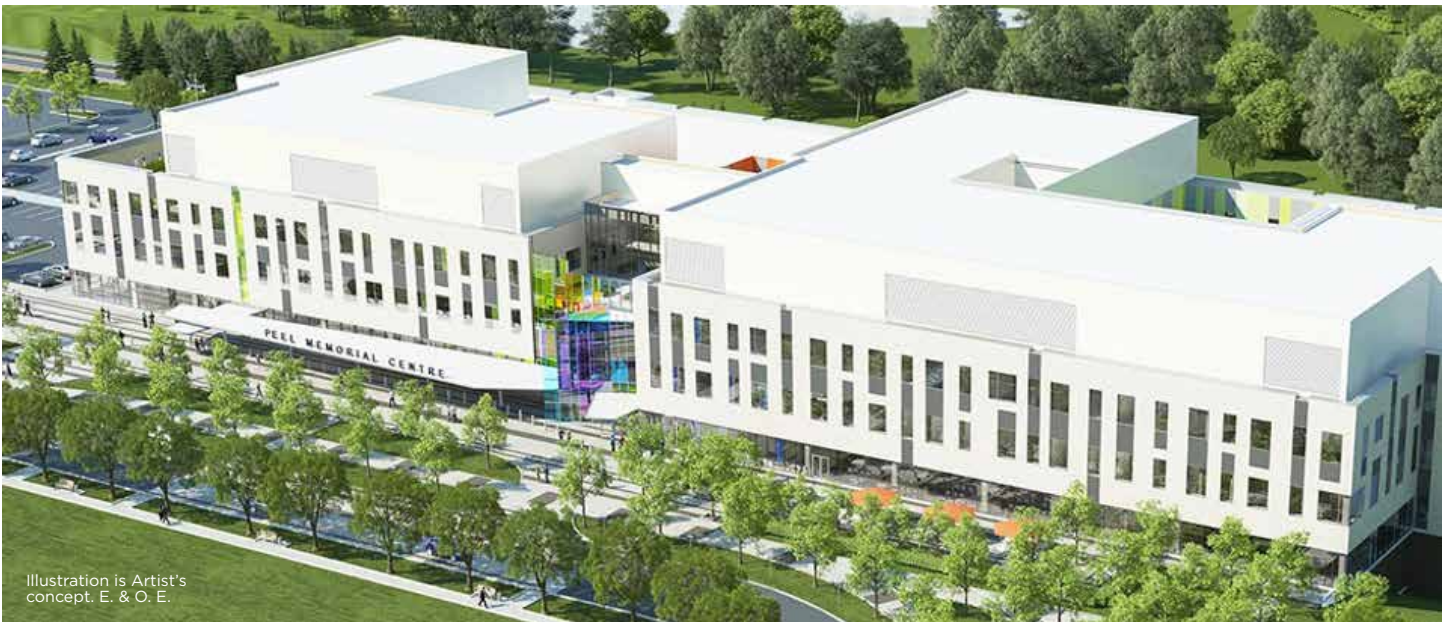
The new Peel Memorial Hospital (Brampton's new second hospital)
